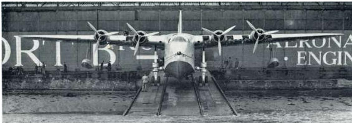
*Canopus, the first of the "C" Class flying boats on the slipway prior to her first flight standing on her beaching gear. Just visible are five open maintenance platforms built into the wing leading edges (four starboard and four port).*
